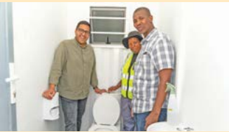
Flush of genius: Cllr Zahid Badroodien, OR Tambo resident Nomandla Mthenjana and Cllr Kayaletu Gxasheka (ward 89 councillor) posing at one of the newly installed toilets that are full-flush, though not dependent on the City's sewers or power grid.
